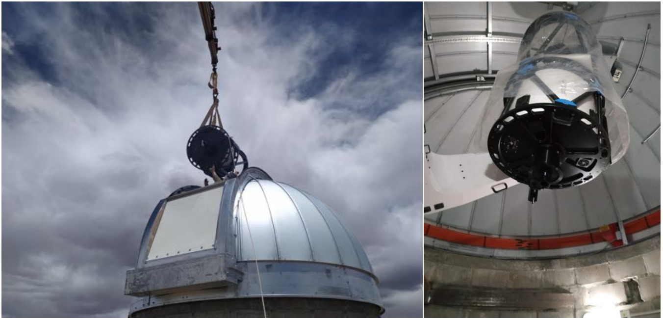
Left: Placing the telescope inside its dome at Cordón Macón. Right: Ready for observations.
