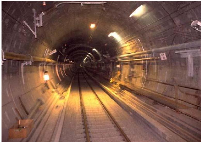
Figure 2.1. Rail tunnel with a precast segmental lining ([www.railway-technology.com](http://www.railway-technology.com))
