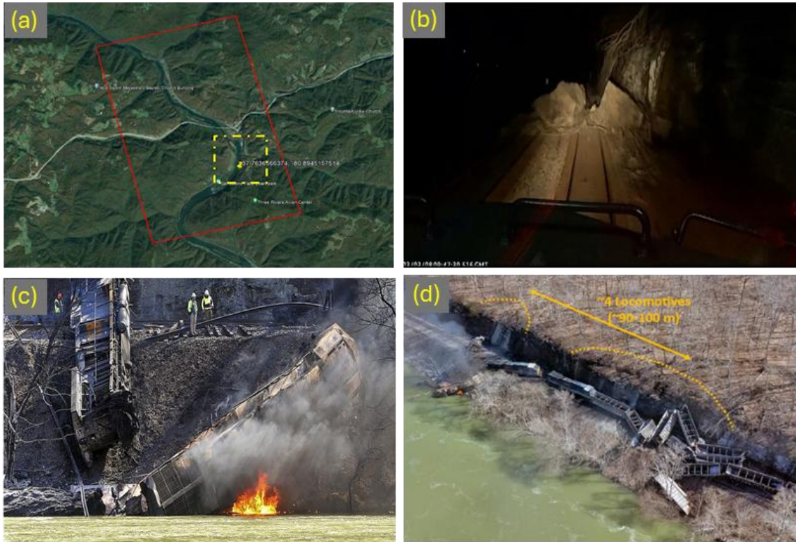
Figure A.39 (a) Incident site; (b) Derailment; (c) Locomotive view of rockfall; (d) Two distinct slope failures ~100 m apart.
