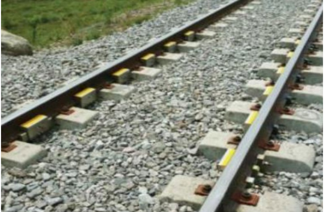
Figure 6: Wheel Impact Load Detectors (WILD) field installation.
