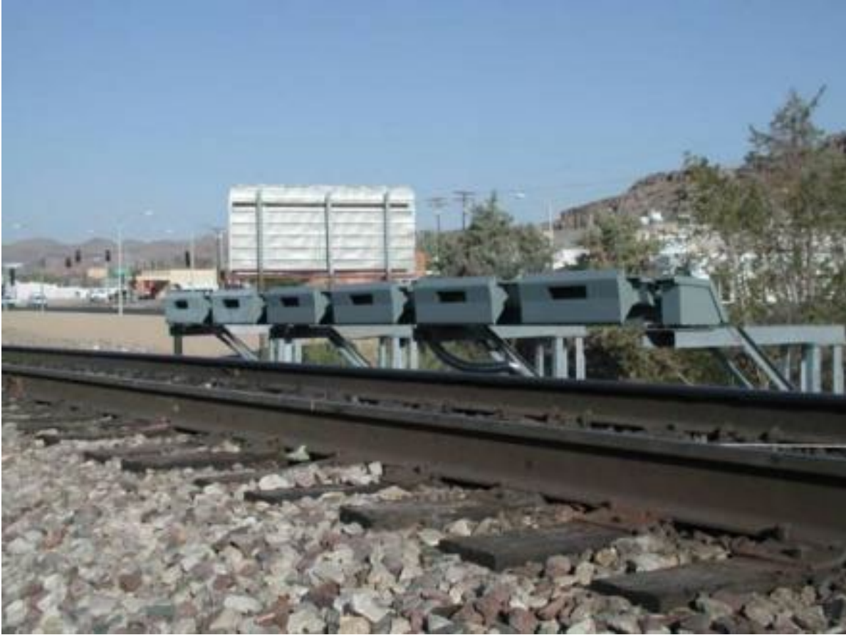
Figure 5: Track Acoustic Detector System (TADS™) at rail side [1].
