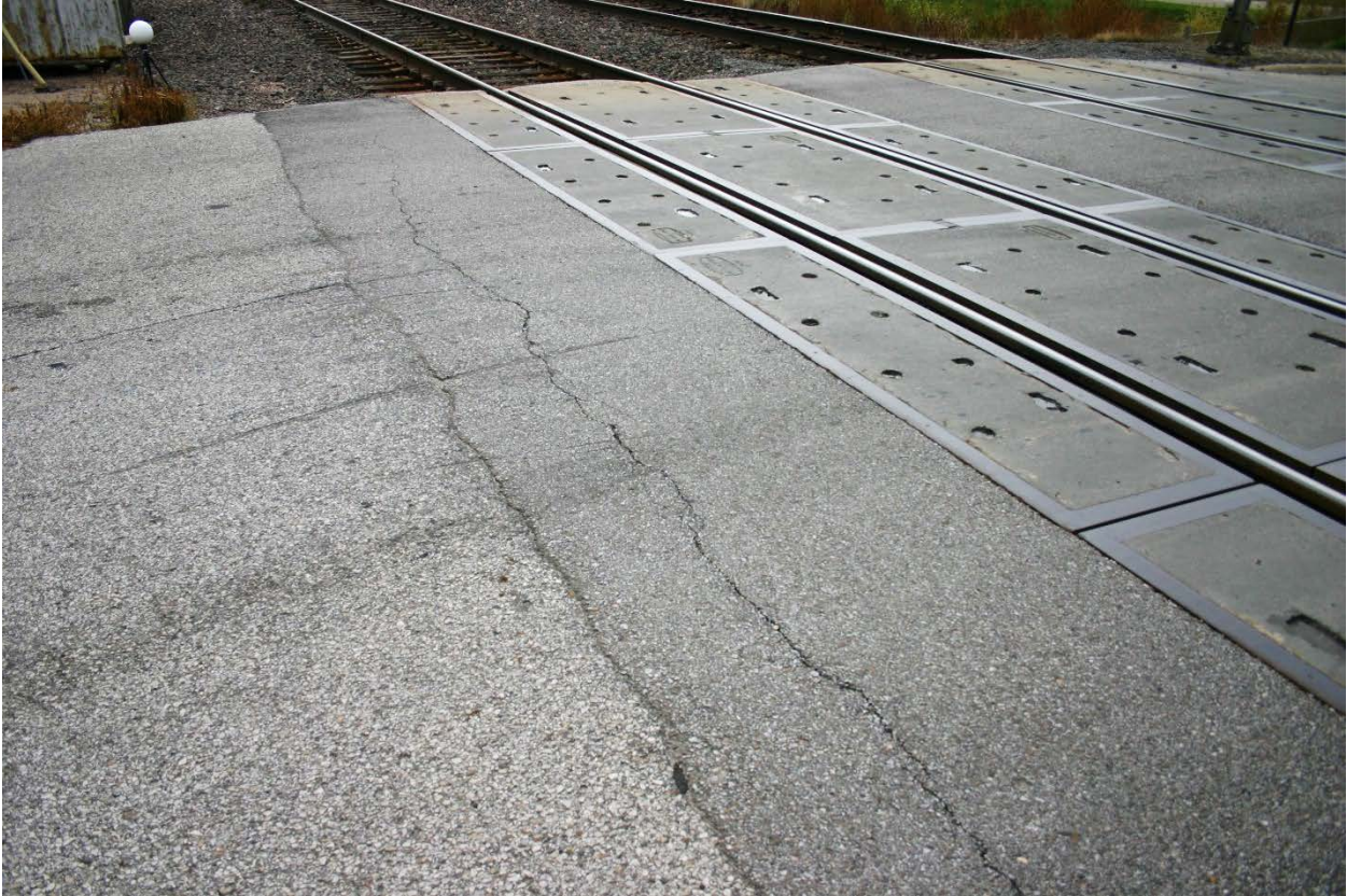
Figure 102. East Approach of Crossing 816134F with Scrape Marks on the Asphalt, Close Up
