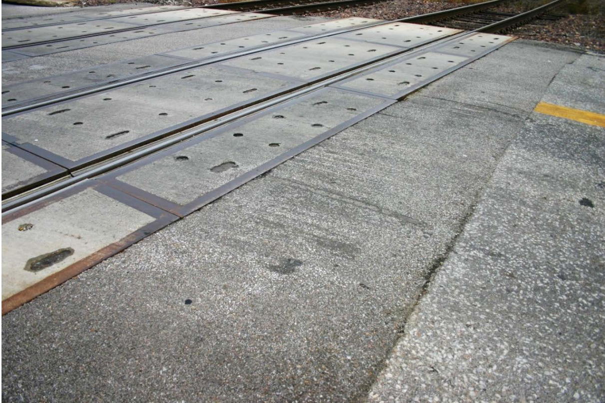
Figure 95. East Approach of Crossing 817405M with Scrape Marks on the Asphalt, Close Up
