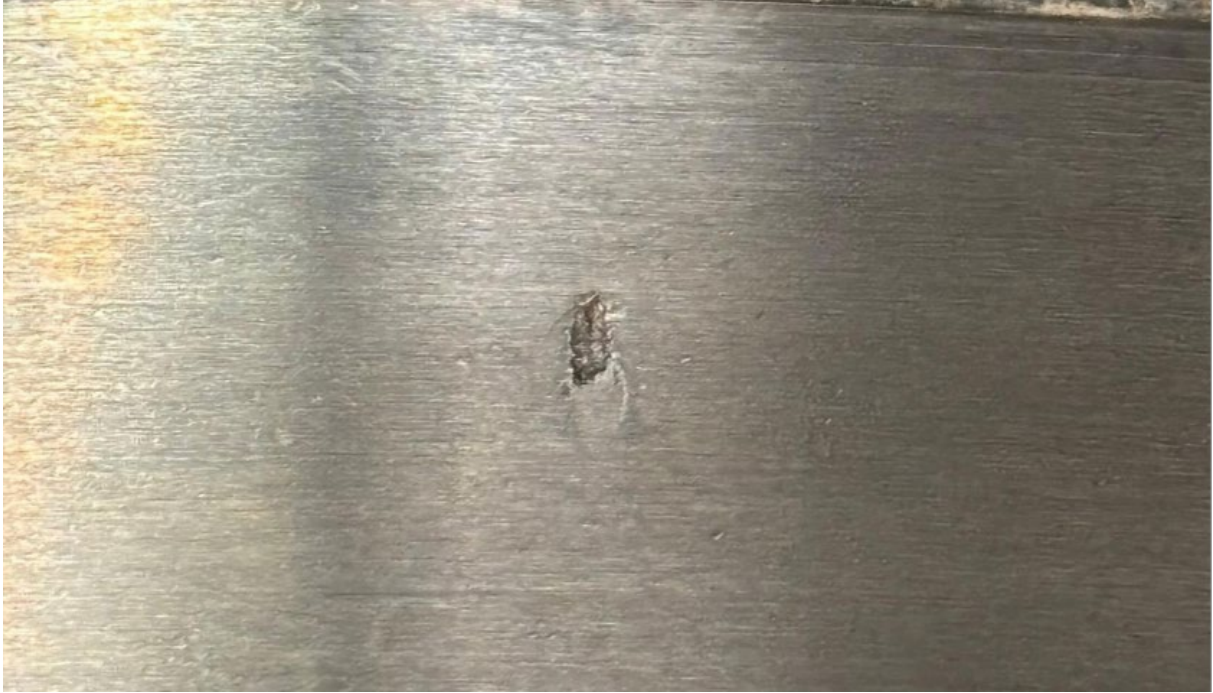
Figure 45: Close-up of small spall on R2 IB cone raceway
