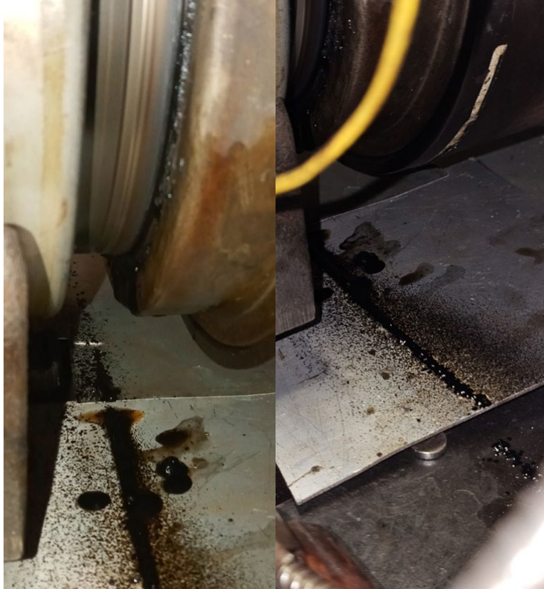
Figure 10: Pictures of grease accumulation below the inboard (IB) seal of bearing L4
