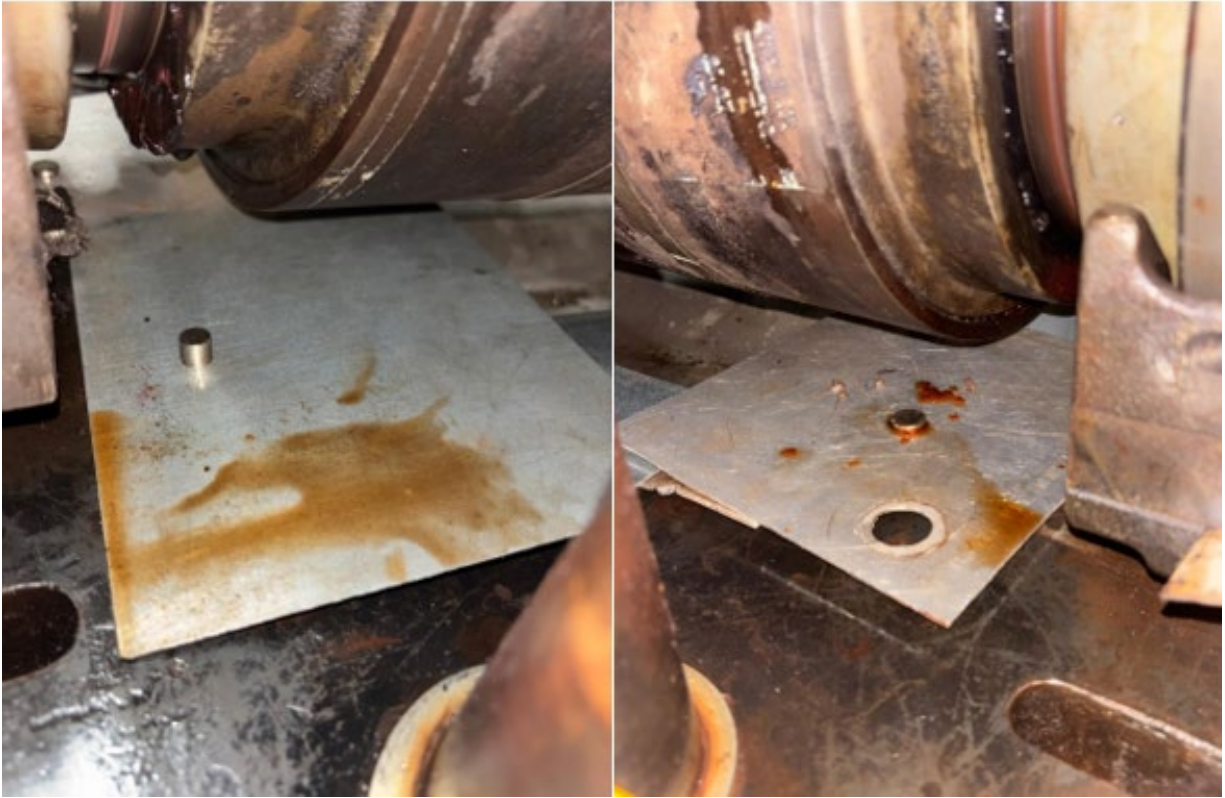
Figure 39: Leaked grease accumulation on IB (L2) and OB (R2) sides (12/30/2024)
