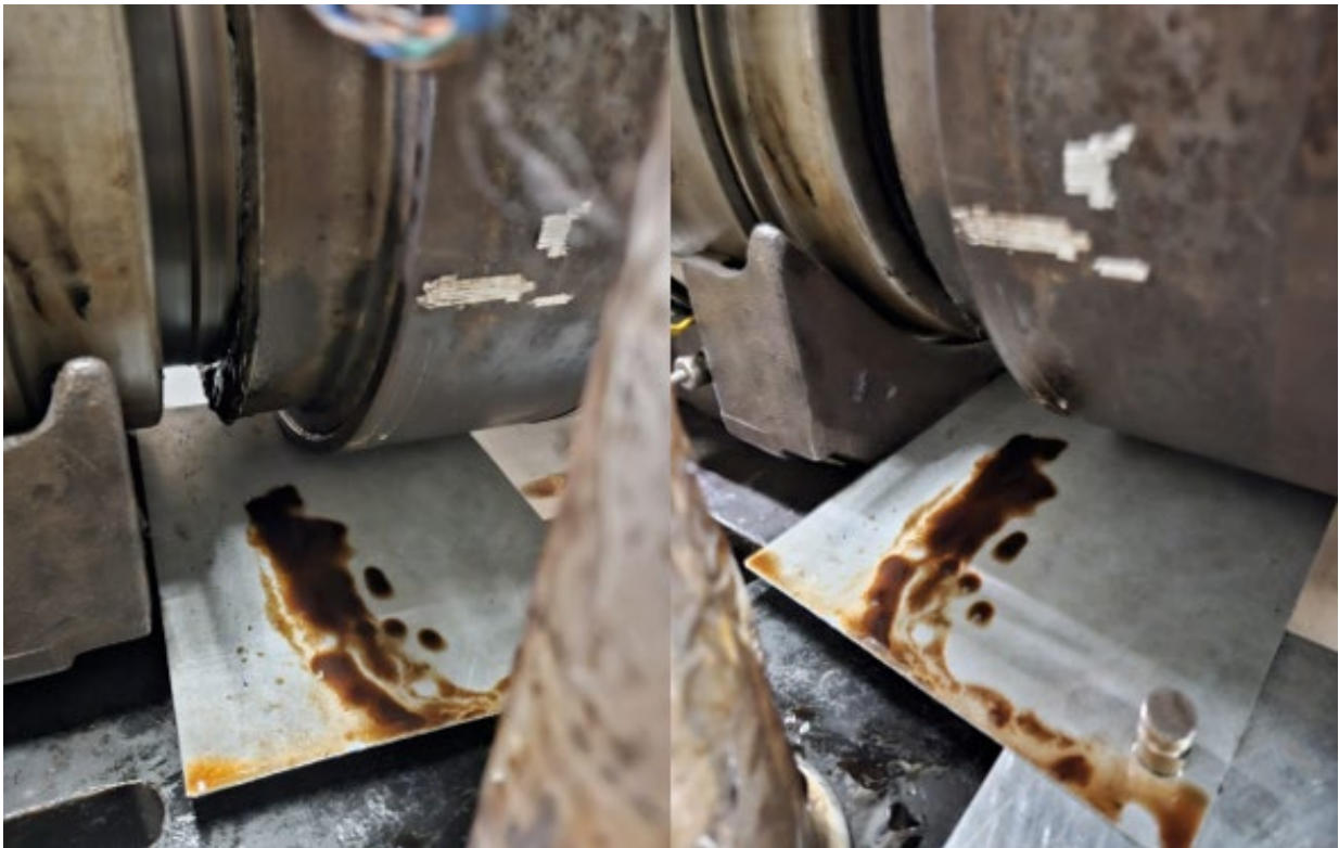
Figure 36: Leaked grease accumulation on IB side of Bearing L2 (12/09/2024)
