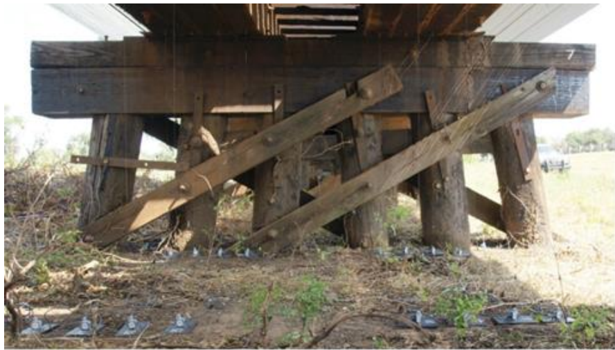
Figure 2: String Potentiometer Setup under Span 7
