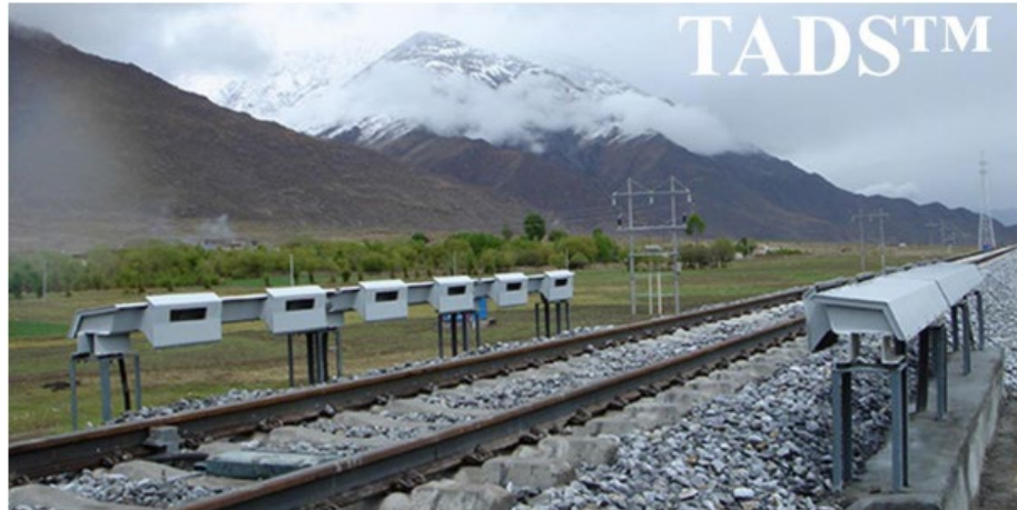
Figure 6. Trackside Acoustic Detection System (TADS™) site [15]
