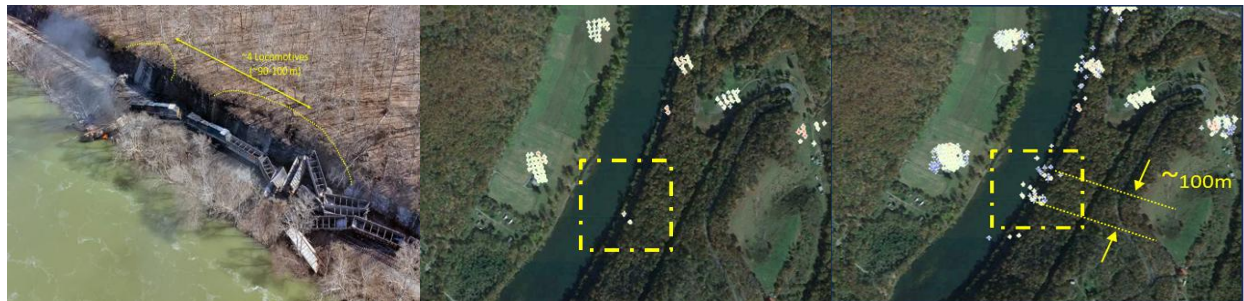
Figure 2 Implementation Example Site 9, Class C, 15 month monitoring before the event: (a) Aerial image of rockfall showing two failure areas 100 m apart; (b) PSInSAR without MTSS deformation map fails to identify potential for failure initiation; (c) PSInSAR with MTSS deformation map clearly identifies potential for failure initiation in two areas 100 m apart at least one month before the event.
