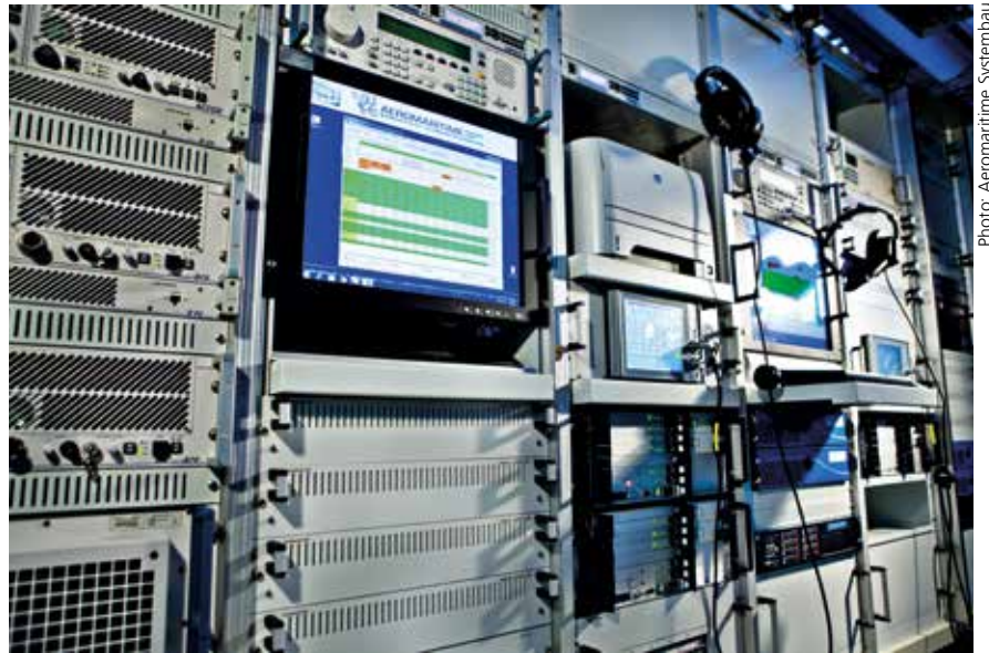
Photo: Aeromaritime Systembau
