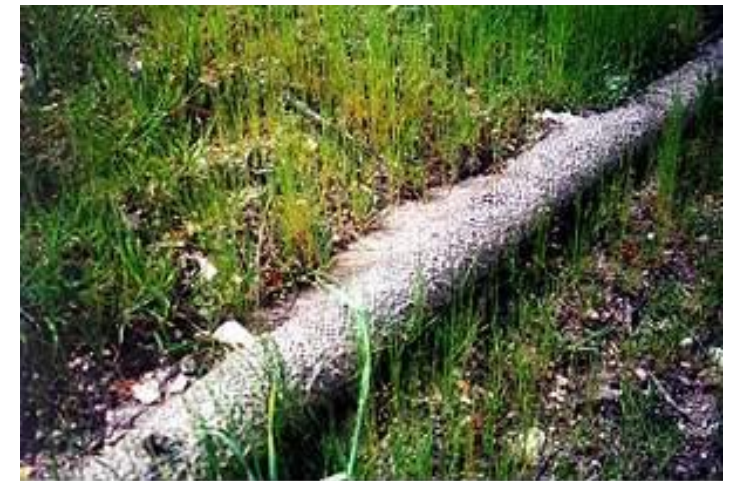
Brush barriers trap sediment and remove pollutants from stormwater
