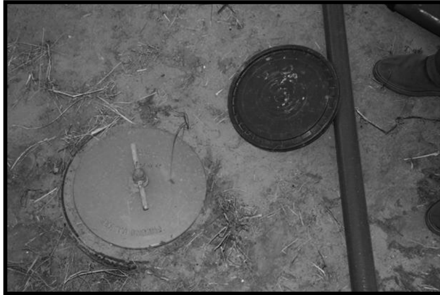
Figure 4.6 Breather valve or pressure valve, Terra Preta Farm Rogers Road Location in Edinburg TX. Picture Courtesy of Professor Roseann Bacha – Garza
