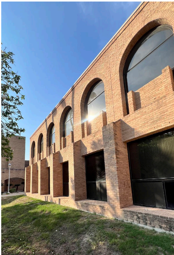
EEDUC Building A
