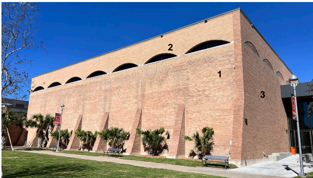
EHPE1 Fieldhouse by Kenneth Bentsen 1972 showing 3 stages of brick repair – 1: Original St. Joe Brick; 2: First repair, date unknown; 3: 2026 facade replacement & repair.
