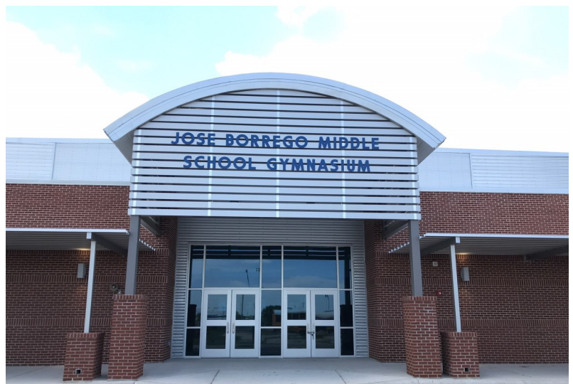
The Jose Borrego Middle School Gymnasium in Monte Alto, TX.
